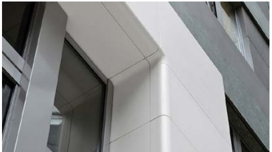
One of the most important features when using HI-MACS® on a façade is its ability to create round corners.
