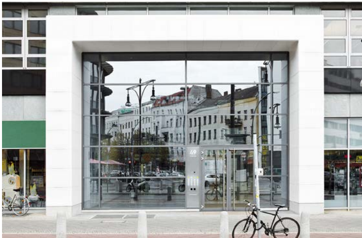
During the day, the lighting technology is invisibly hidden and protected by the robust HI-MACS® surface.
