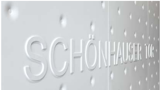
Effectively animated outside, inside a clear design of dots and letters milled out by using the CNC technology.
