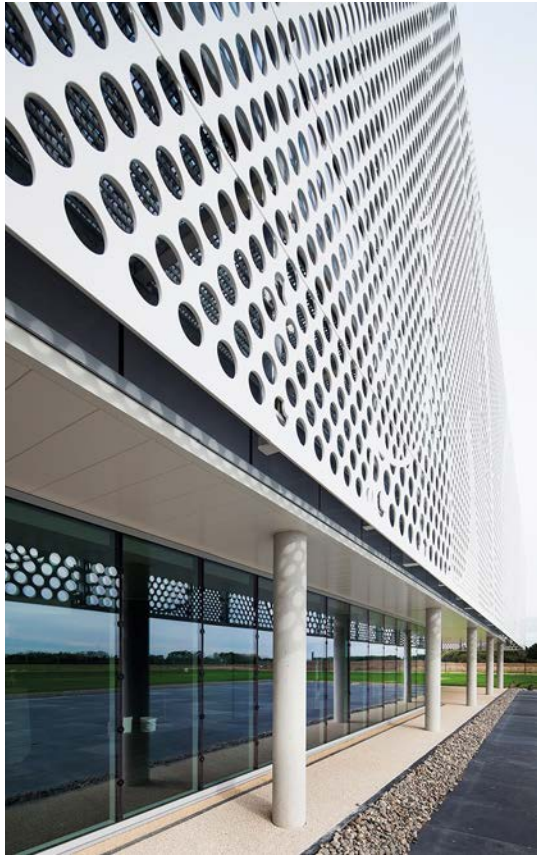
Design: PAD Architectes for BERI 21 | Fabrication: LCCA | Photo: Mathieu Ducros
