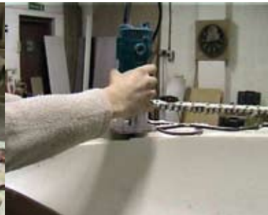
Seam preparation by trimming
